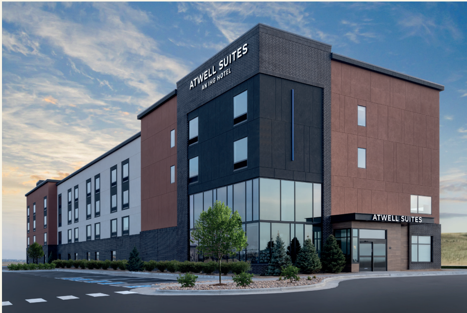
Two-Story, End-Loaded Lobby
